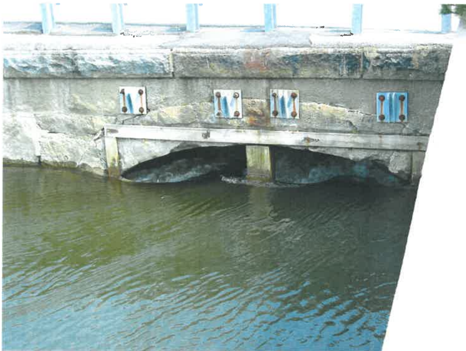
Photo 11. Timber supporting beam on estuary side of bridge.
