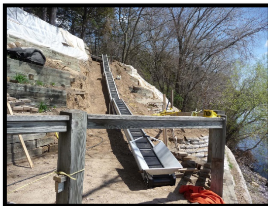
Photo 3 – Example of conveyor belt system that would likely be used to remove excavated material
