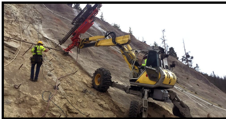
Photo 1 – Spider excavator installing soil nails
