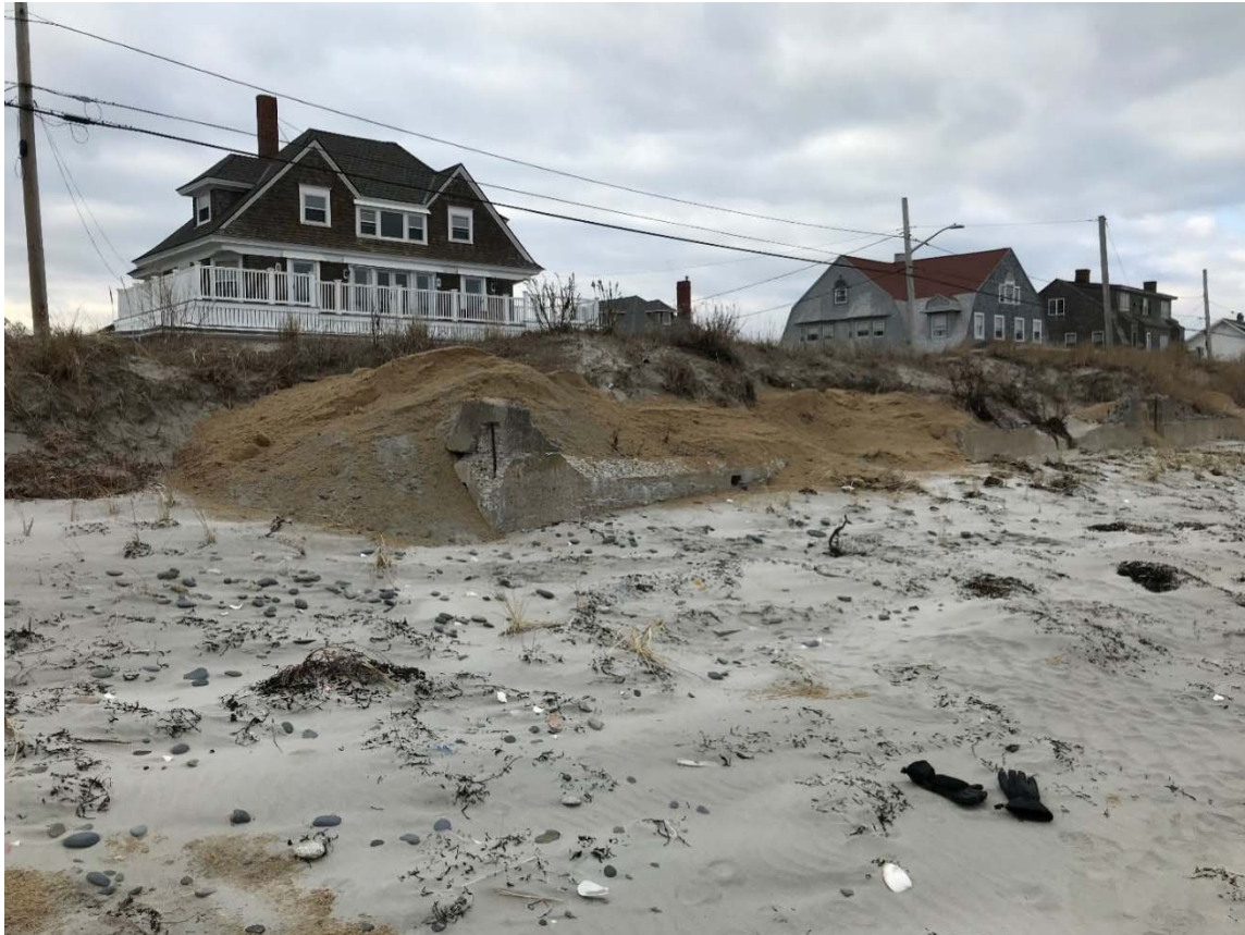
Area 8", more sand was added, Jan. 2019
