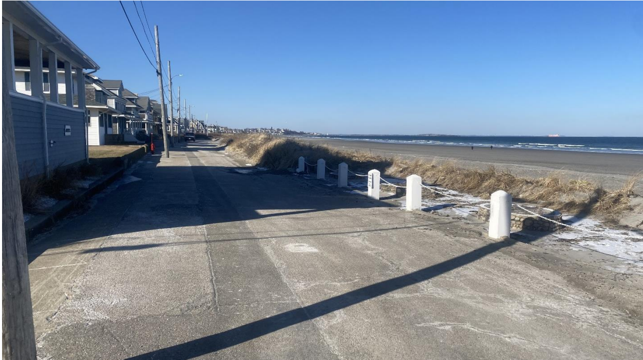
Figure B-13. View north of gap in the primary dune adjacent 33 Malta Street, showing altered dunes to the north.
