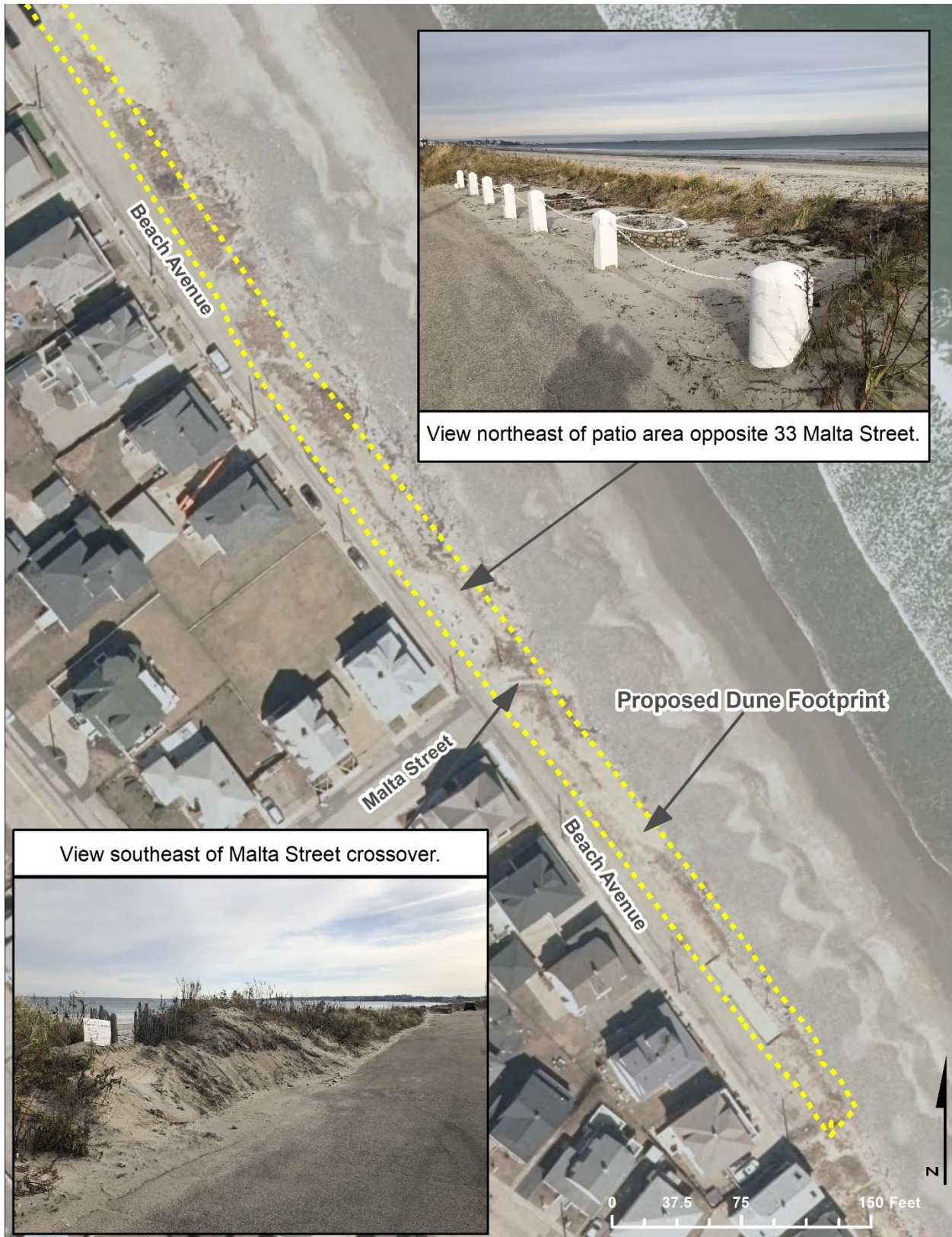
Figure B-3. MassGIS 2019 aerial imagery and site photos of the southern portion of the project locus adjacent to the intersection of Beach Ave and Malta St.
