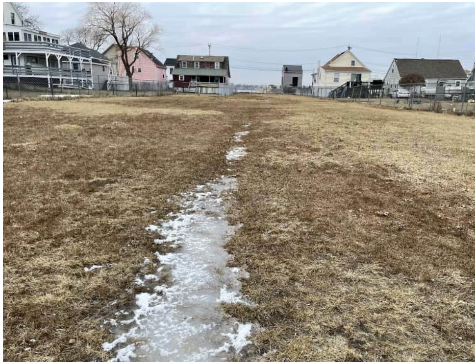
View of frozen water behind the basketball court—facing west.
