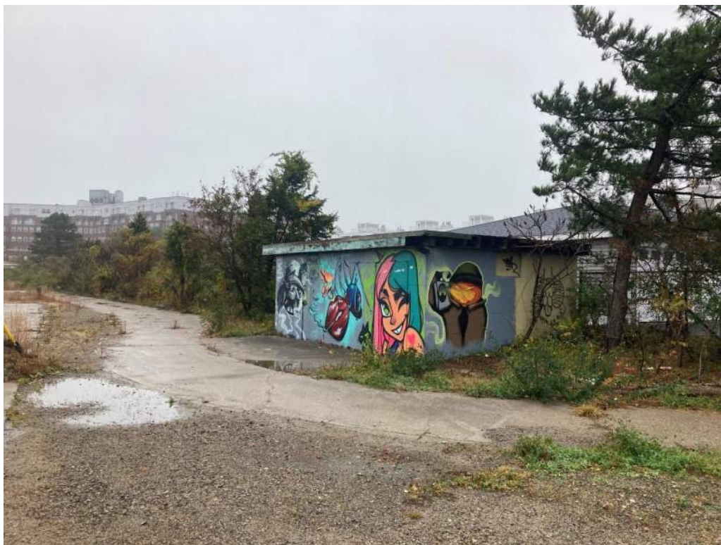
Photograph 4: Structure at South end of 0 GW Blvd Parcel
