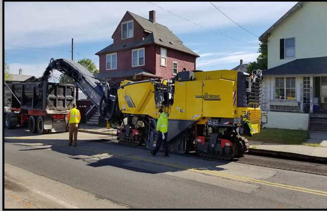
Mill and Overlay
