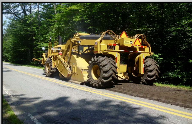
Full Depth Reclamation
