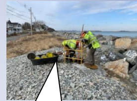
"Fishing" to retrieve PIGS at end manhole
