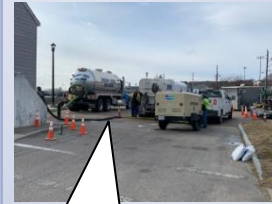
Pump Station bypass
