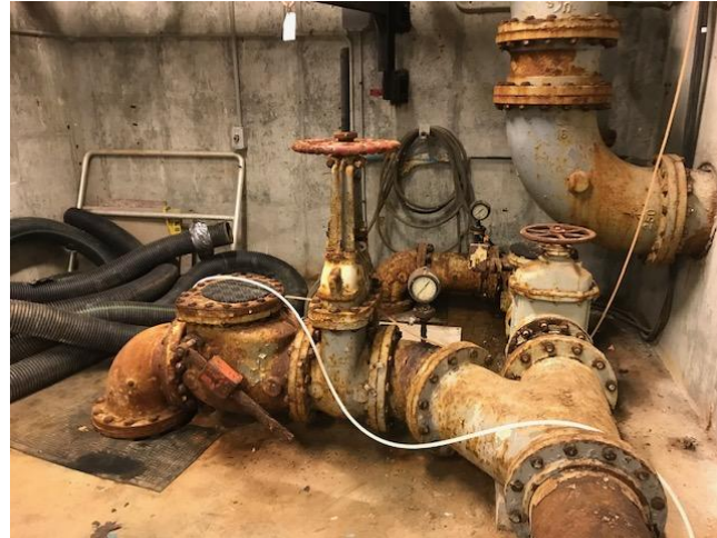
The Effluent Pump Room valves are severely corroded and in need of replacement
