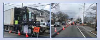
The felt/resin liner is pulled through the existing pipe and steam is used to cure the liner.
