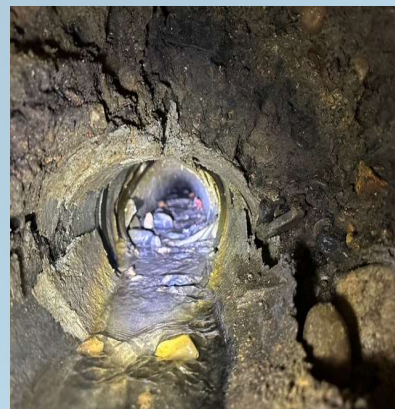
Collapsed pipe restricting flow by more than 50%
