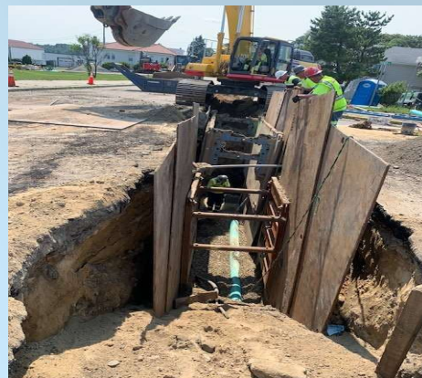
Sewer pipe replacement across Nantasket Avenue
