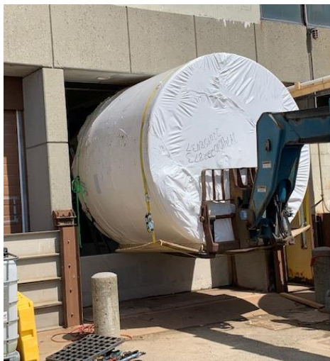
Putting a round peg into a square hole. Tight fit placing one of the sodium hypochlorite tanks into the control building.
