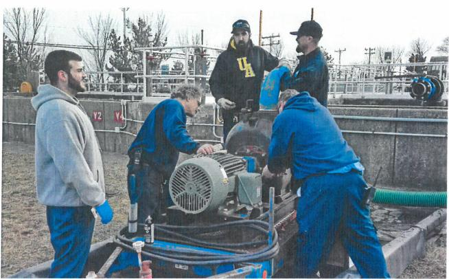
Staff made changes to a backup process pump so it can be used to send mixed liquor suspended solids directly to a chlorine contact chamber if necessary during a high-flow storm event.
