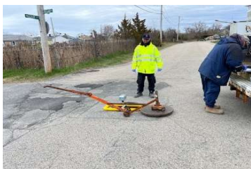
Acoustic monitoring from manhole to assess if sewer needs cleaning
