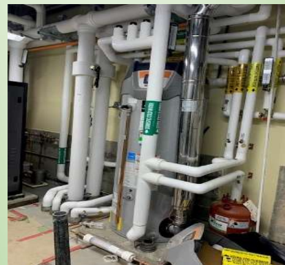
Below - New Boiler Room and Piping
