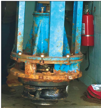
Pump being removed to be rebuilt
