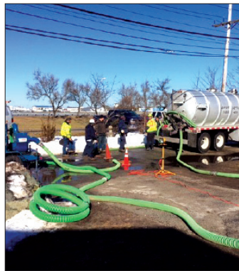
Surface bypass pump to divert water
