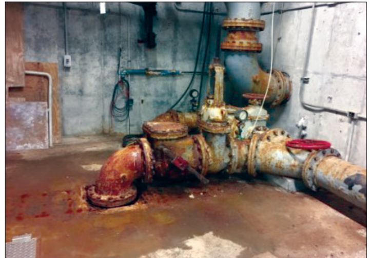
40 years of corrosion is taking a toll on all of our piping
