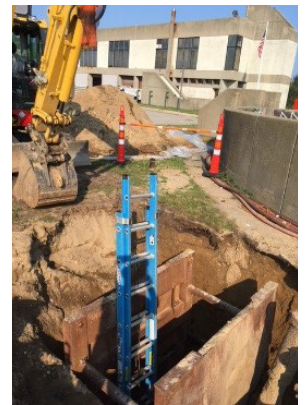
Valve Replacement Excavation
