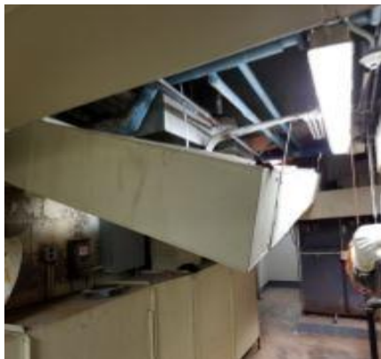
Failed HVAC ductwork in basement
