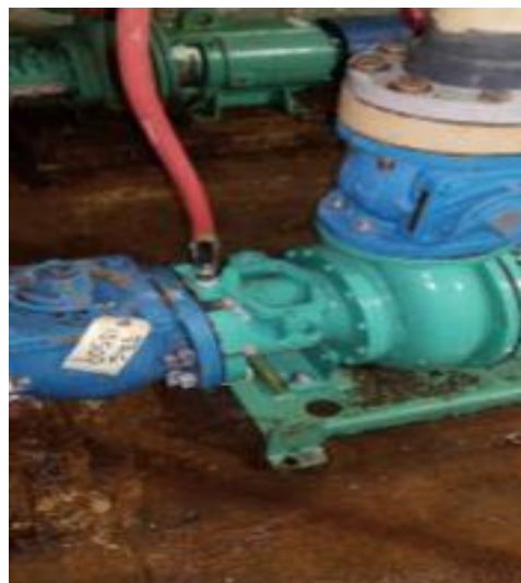
Polymer injection point into sludge feed line
