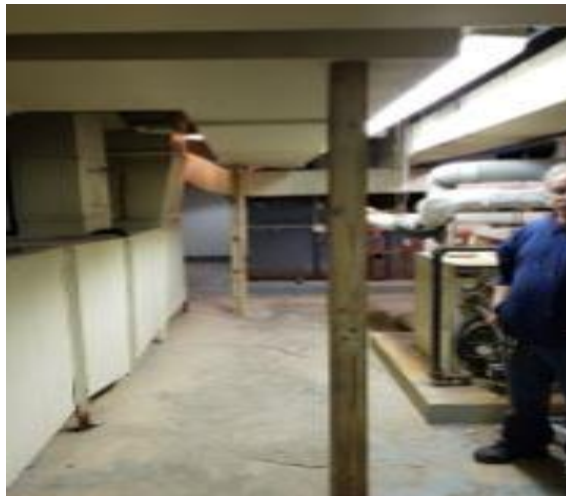
Temporary supports for HVAC ductwork to correct an unsafe condition
