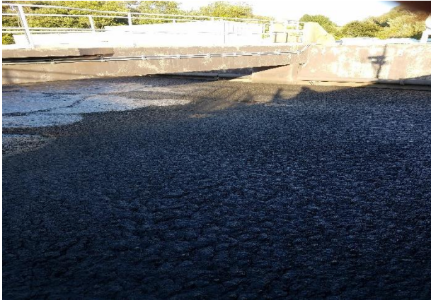
Aeration tank #1 [dark foam – high solids]
