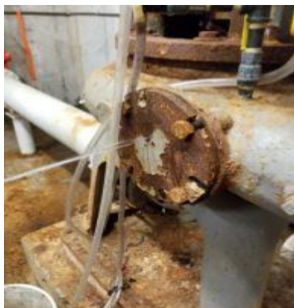
Cleanout cover – repaired with ceramic coating
