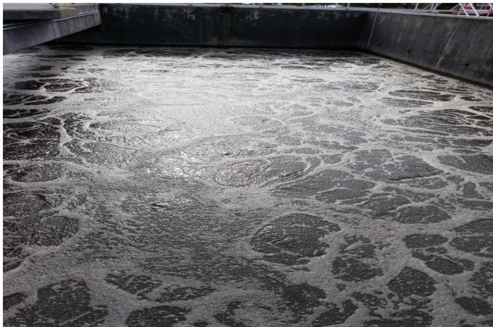
Aeration Tank – diffused air system
