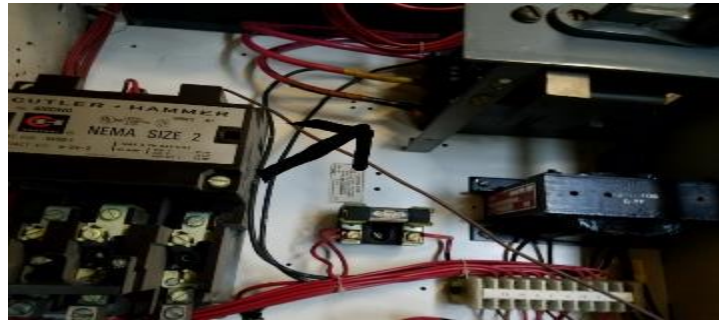
MCC bucket with motor starter with burnt wire
