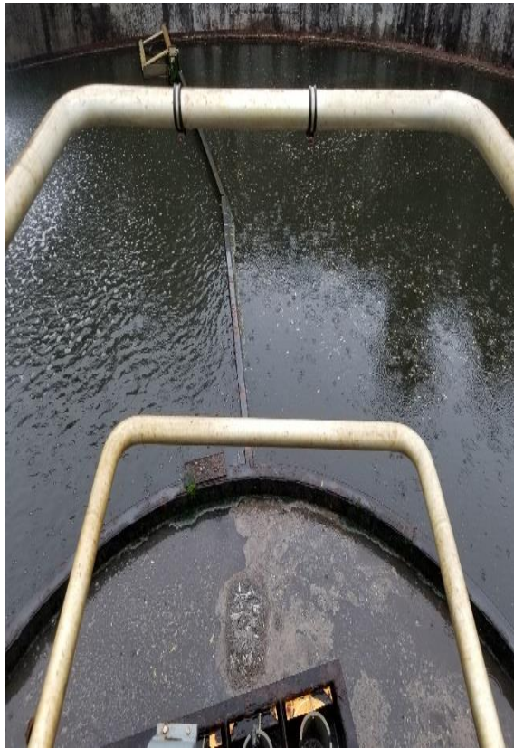
Secondary Clarifier effluent
