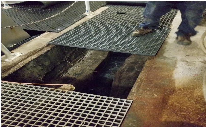
Influent Headworks – parshall flume in channel under the grating
