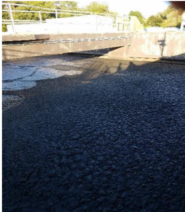
Aeration tank #1-darker foam – high solids
