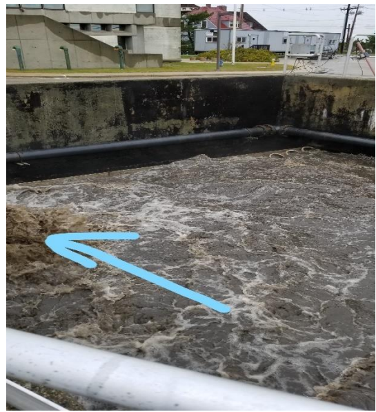
Tank 3 – while in service with broken diffuser piping – blowout of air
