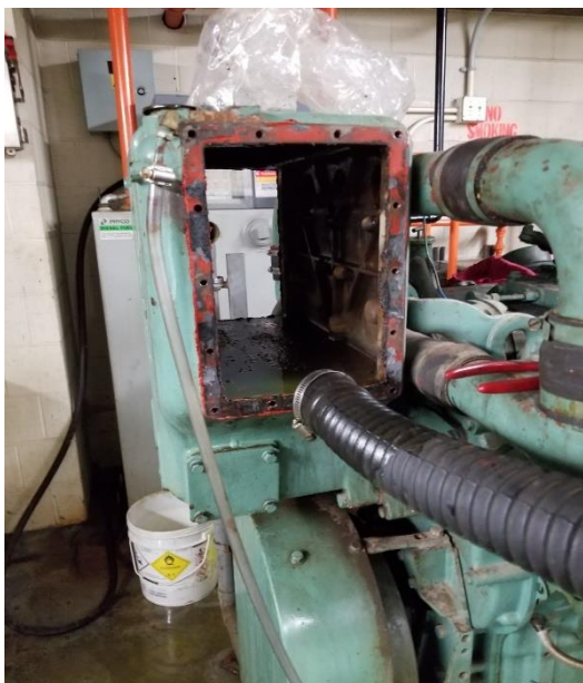
520KW unit – heat exchanger removed for repair
