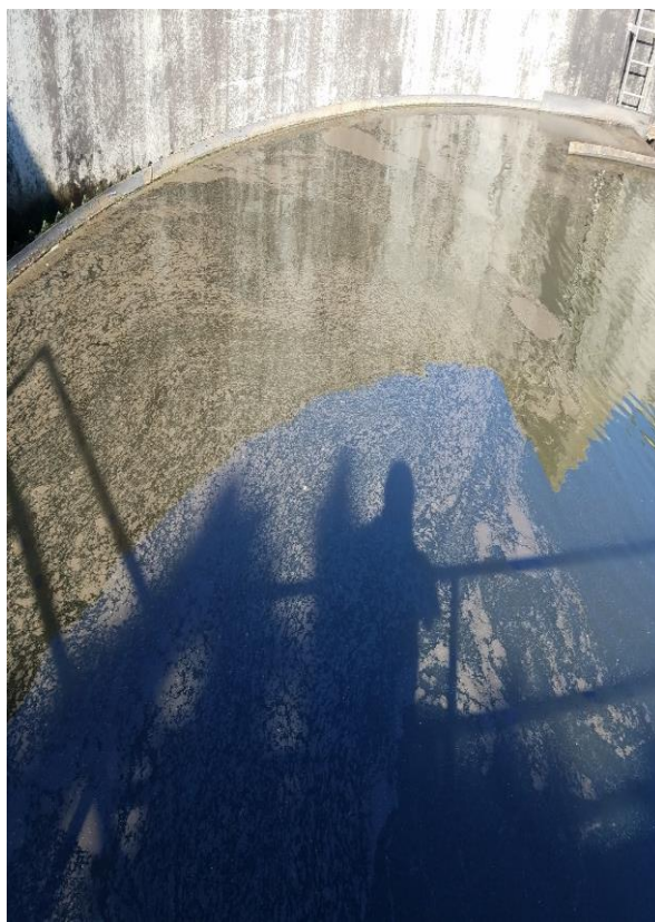
Secondary Clarifier increased floating solids
