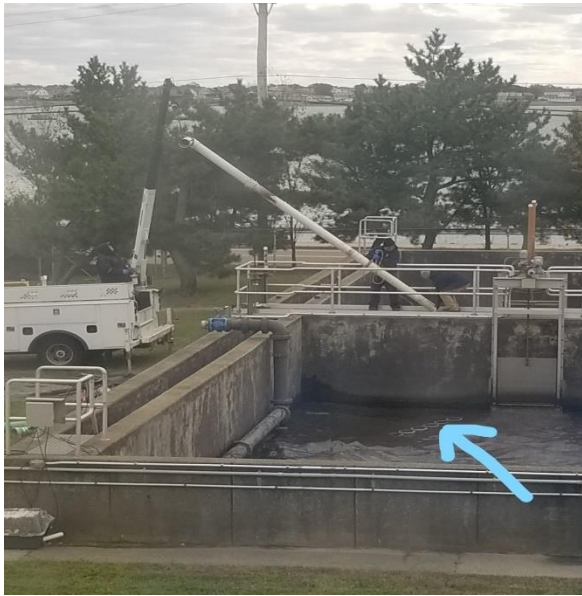
Tank 3 – ready to pump down – broken diffuser in background
