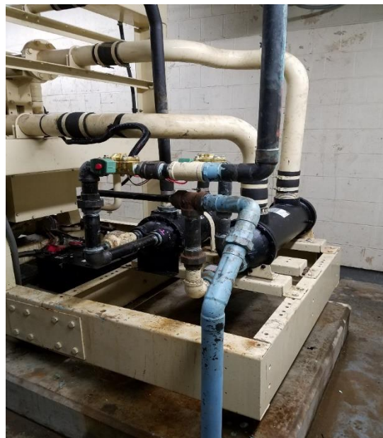
750KW unit – two new heat exchangers [black]
