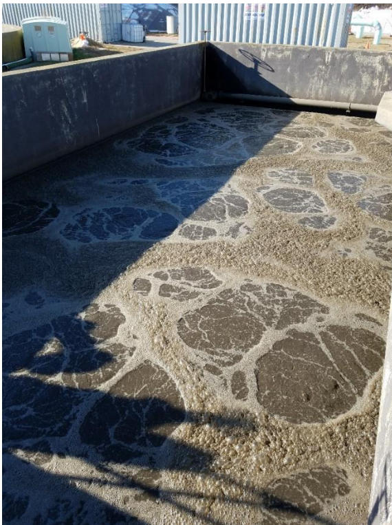
Aeration Tank #1 - increased foam/solids
