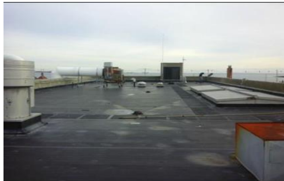
Picture of Operations building roof – membrane had a number of tears that were repaired on 11/15/18
