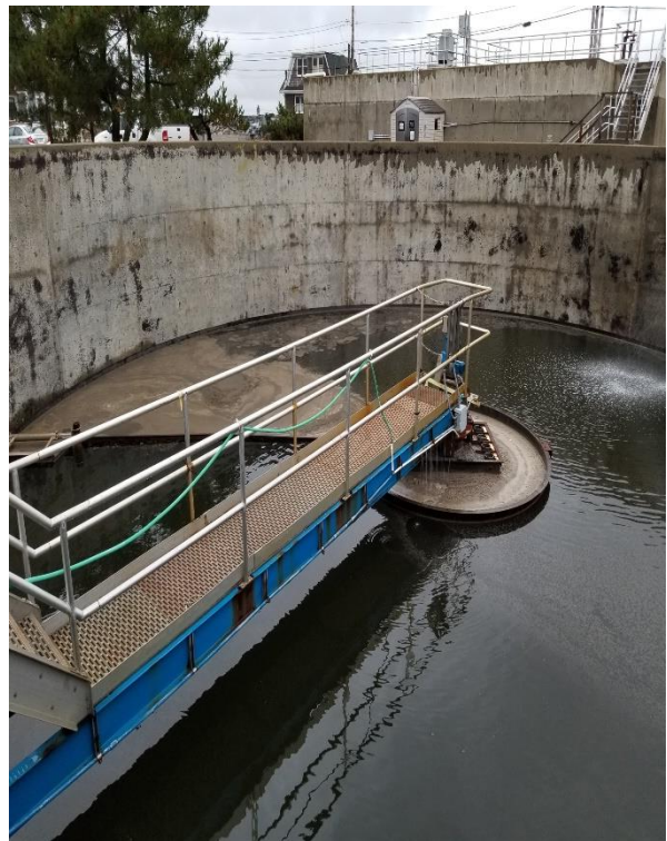
Secondary Clarifier increased floating solids
