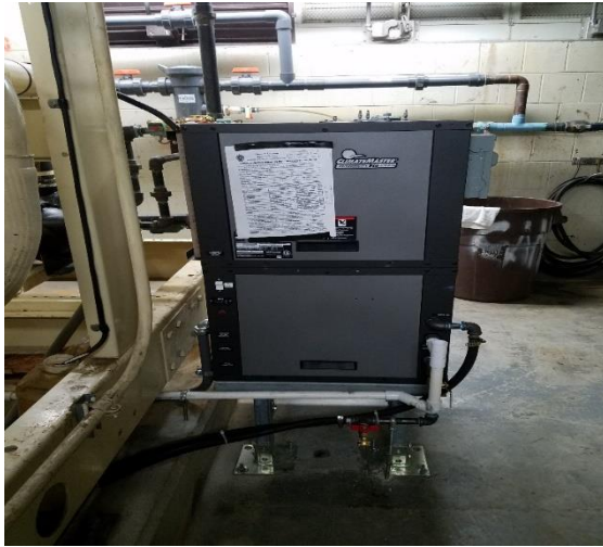
Heat pump that is tied into block heater
