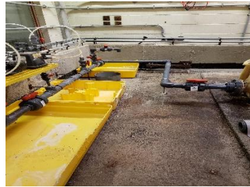
Repaired manifold piping from Tank #2
