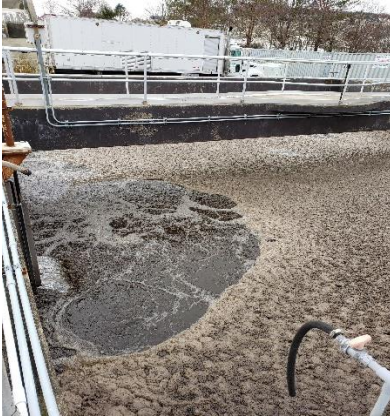
Aeration tank #1- less & lighter foam
