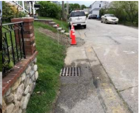
Downstream catch basin that was cleaned out
