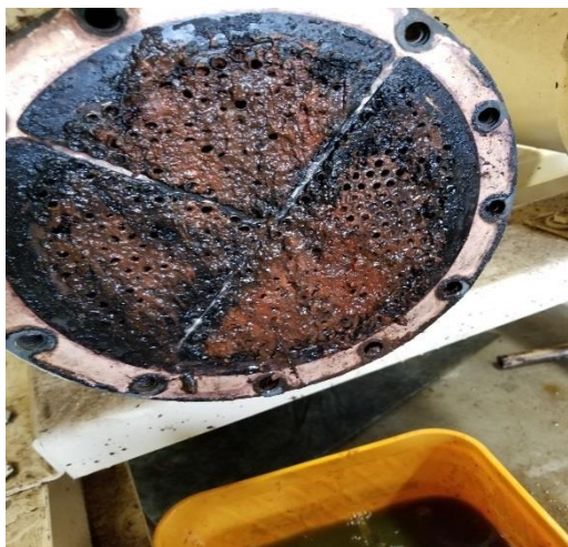
Gen #1 internal blockage and corroded tubes
