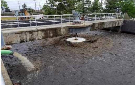
Aeration tank #4 being filled
