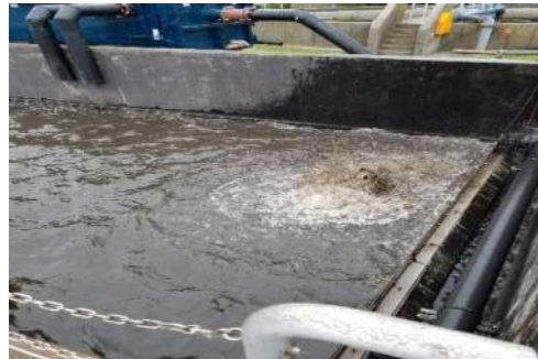
Aer tank #1 grid piping failure
