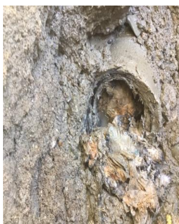
Debris build-up at end of lateral
