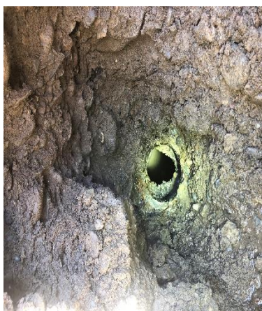
Inner liner from relining project
