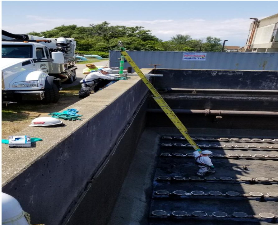
Confined space equipment for permitted access into tank
