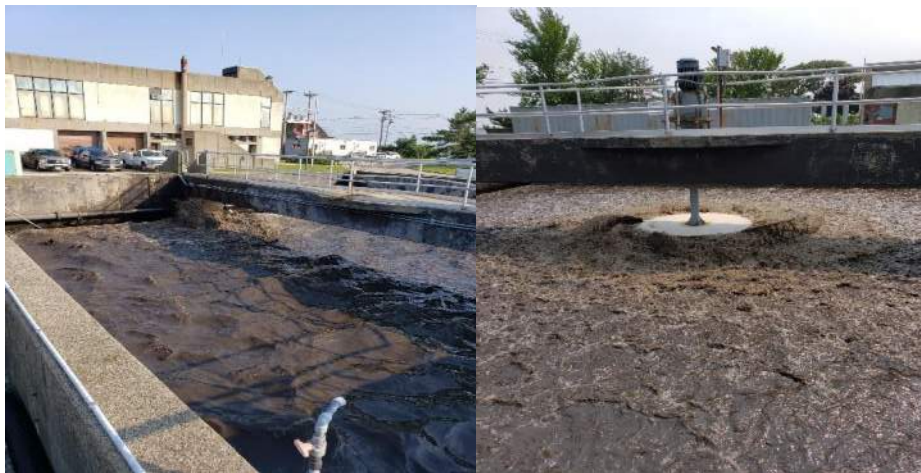
Aeration tank #3 loss of air due to piping failure Aeration tank #2 – mechanical aerator
