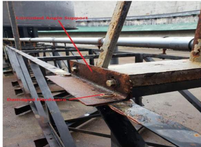
Angle supports on skimmer post are corroded – hardware damaged
