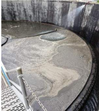
Floating sludge on clarifier surface
