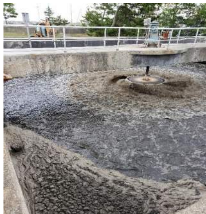
Mechanical aerator – insufficient mixing
