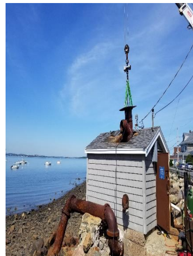
Vertical lift pump being removed
