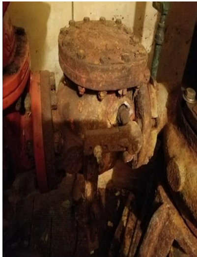
PS 1 pump discharge check valve
