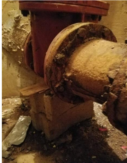
Inadequate pipe support
