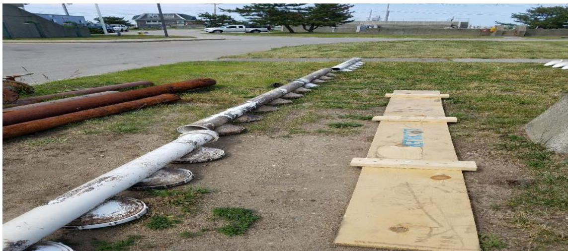
Sections of diffuser piping removed from tank that broke, and new piping installed
