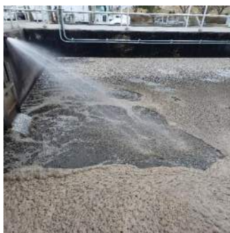
Aeration tank #1- moderate foam
