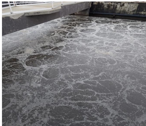
Aeration tank #3 – good solids level & color
