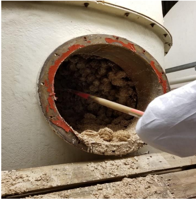
Removal of old scrubber media from vessel
