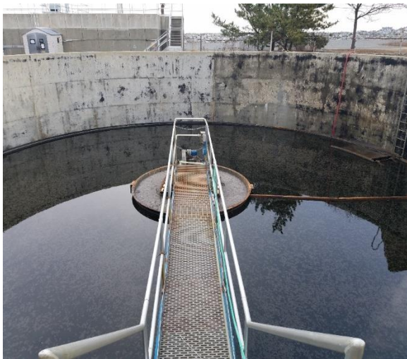
Secondary Clarifier - good clarity & no water spray
