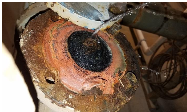
Blockage in header pipe from plant water pump discharge [in sub-basement]
