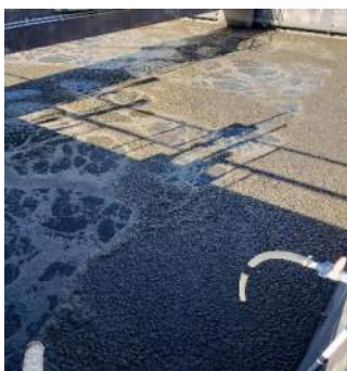
Aeration tank #1- moderate foam
