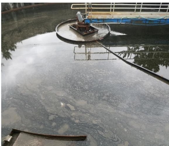
Secondary Clarifier - good clarity & no water spray
