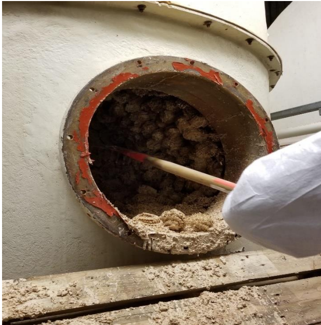
Removal of old scrubber media from vessel
