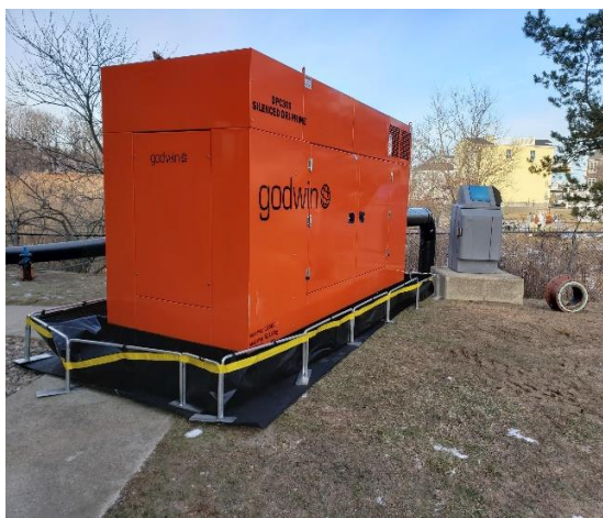
New containment berm in place
