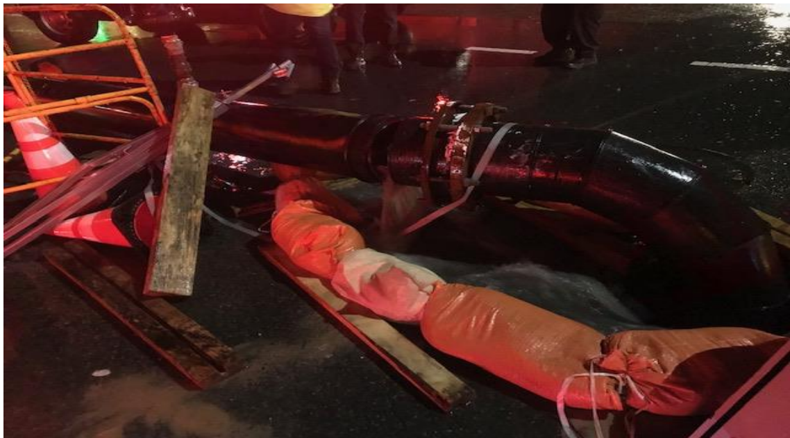
Sandbagging of area of break to divert flow into the manhole
