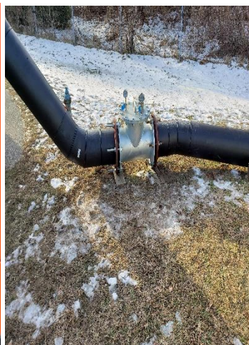
Piping modifications for pump suction and discharge with additional screens, flush connections, and gauges
