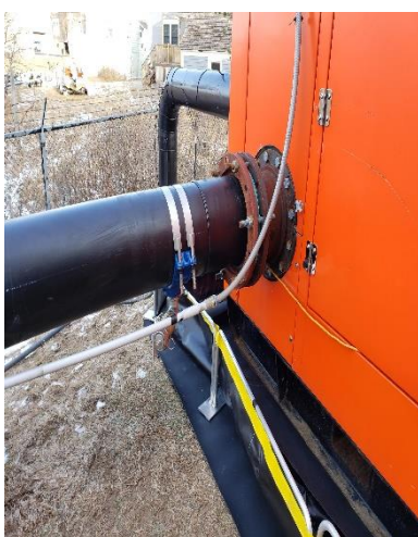
Piping modifications for pump suction and discharge with additional screens, flush connections, and gauges
