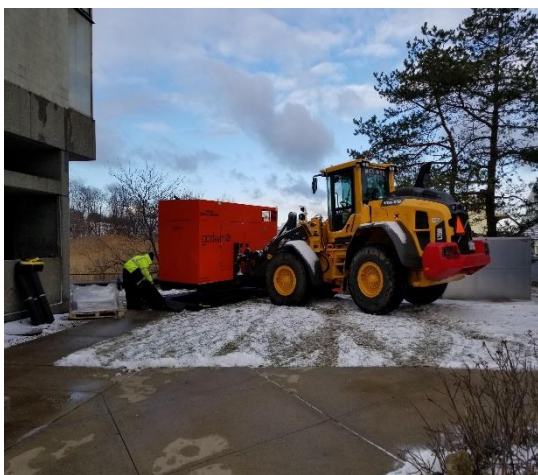
Lifting of Godwin Pump [Aqualine loader]
