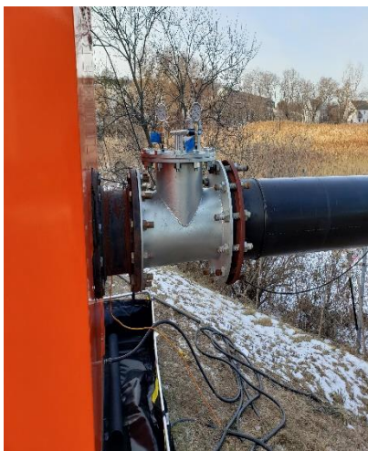
Piping modifications for pump suction and discharge with additional screens, flush connections, and gauges
