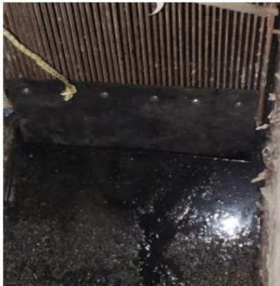
Bar rack in place with rubber seal/extension
