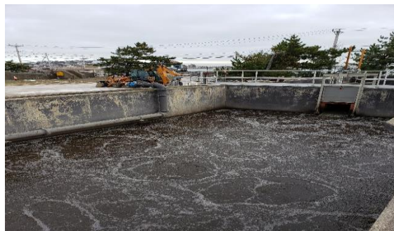
Aeration tank #3 [moderate brown color, no foam]
