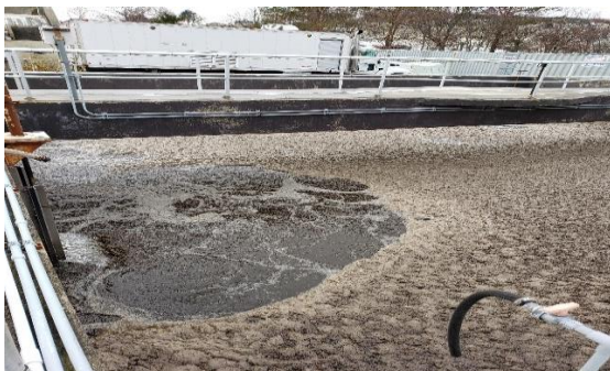
Aeration tank #1- moderate foam
