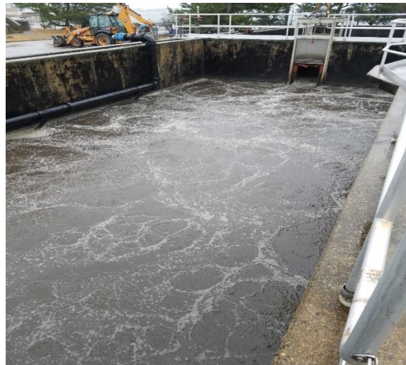
Aeration tank #3 – lower solids levels/better color
