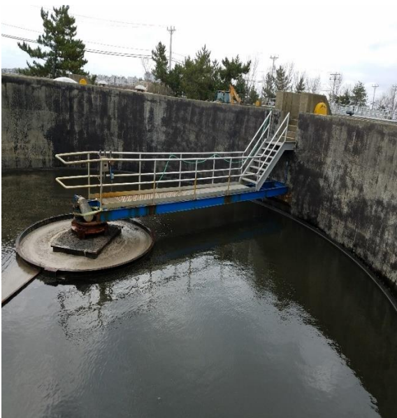
Secondary Clarifier improved clarity
