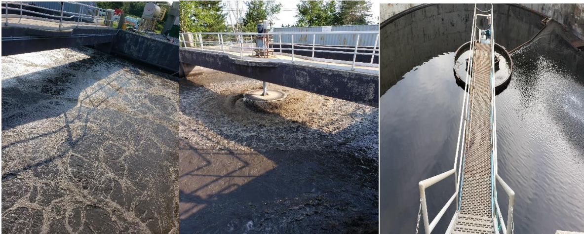
Aeration tank #3 loss of air due to piping failure Aeration tank #2 – mechanical aerator
