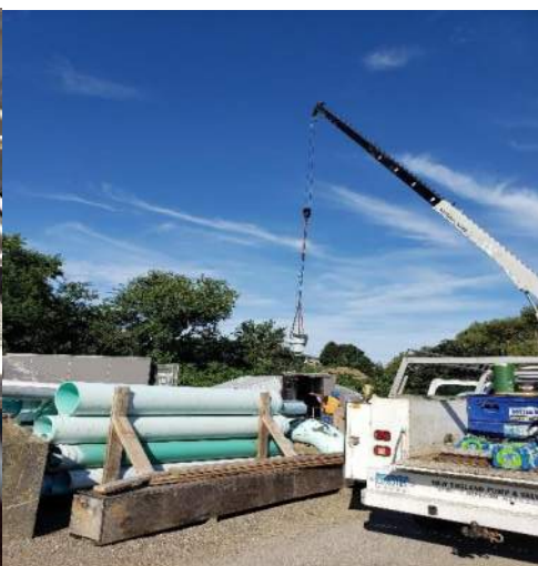
New gear box being lowered into the tank through roof opening
