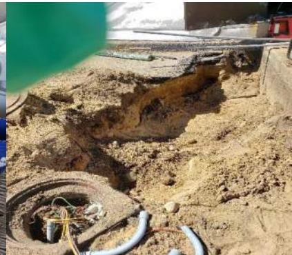
New conduit and wiring for GT #1
