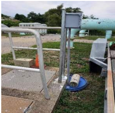
New level probe for SHT2 – junction box
