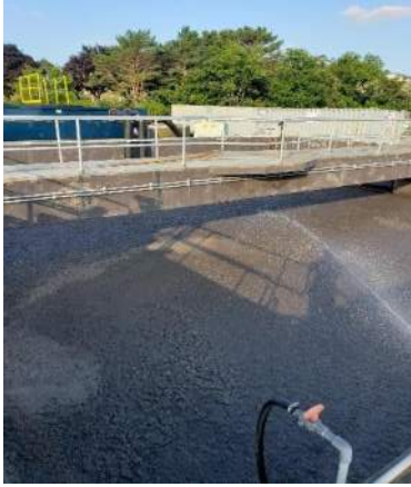
Heavy solids/foam on aeration tank #1
