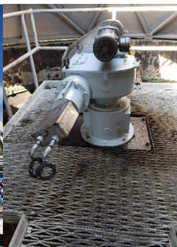
New gear box in place
