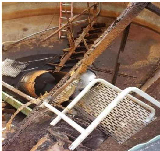
GT #2 – collapsed equipment in tank
