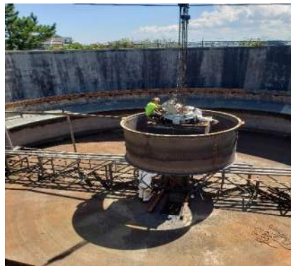
Setting new gearbox in place by Lydon
