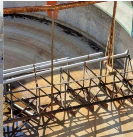
New scraper blades installed
