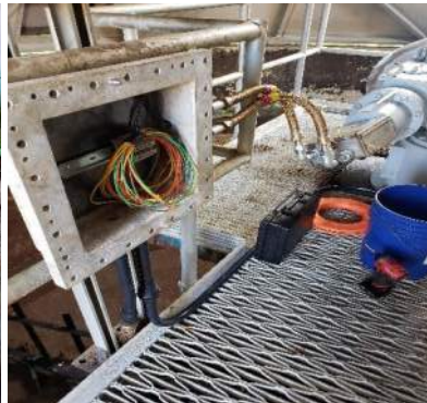
New wiring for GT #1 motor and controls
