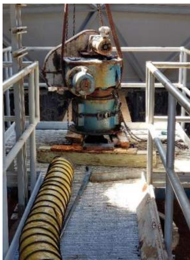
GT #1 – old gear box ready for removal
