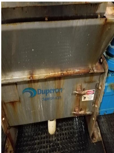
Wash compactor for bar screen
