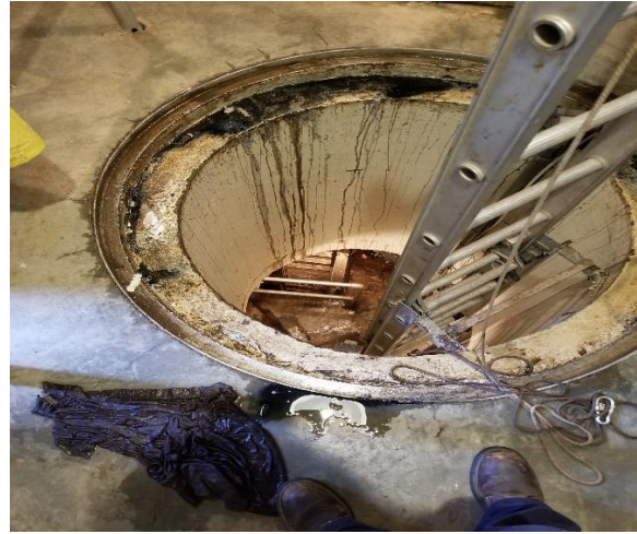
Inside PS1 where leakage flowed due to FM break
