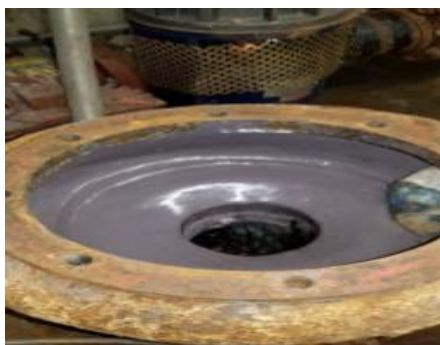
Lining of RAS volute with ceramic putty
