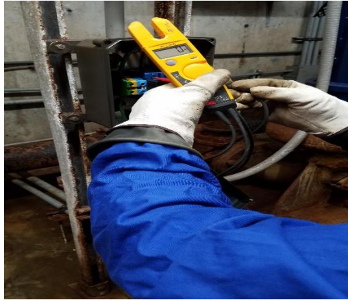
Dave W performing zero voltage check for LOTO for RAS pump
