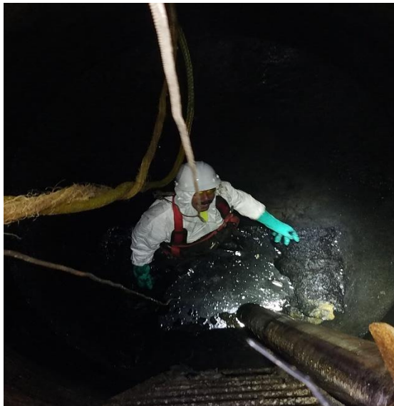
Jody S showing corroded and broken pump suction pipe
