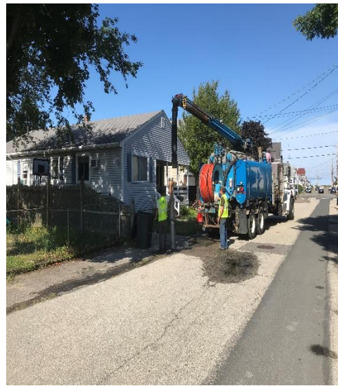
Nantasket [green dots] show catch basins cleaned out GMPS vac truck cleaning the catch basins Nantasket Ave & E street
