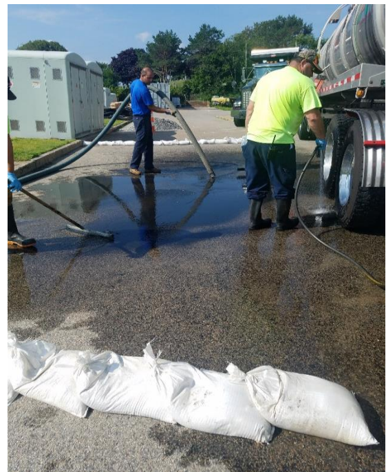
Used sand bags to contain spill and vacuum Up all washdown water.
