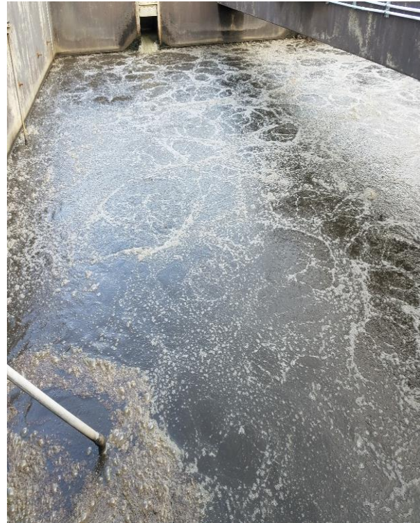
Normal air distribution pattern – repaired aeration basin #1
