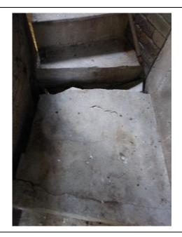
Photo of a missing portion of a stair platform.
