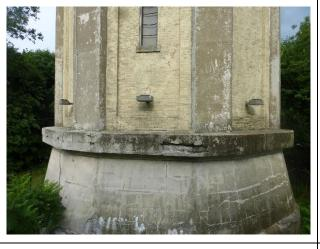
View of the reinforced concrete column and coated concrete brick masonry infill between the columns.
