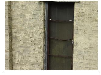
Typical view of a dilapidated window possibly original to the construction of the water tower.
