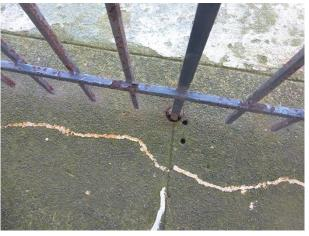
Photo of the base of the railing system with an unsealed hole through the concrete deck at the observatory level.
