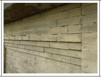
Photo of failed and eroded mortar joints below the upper decorative concrete band.
