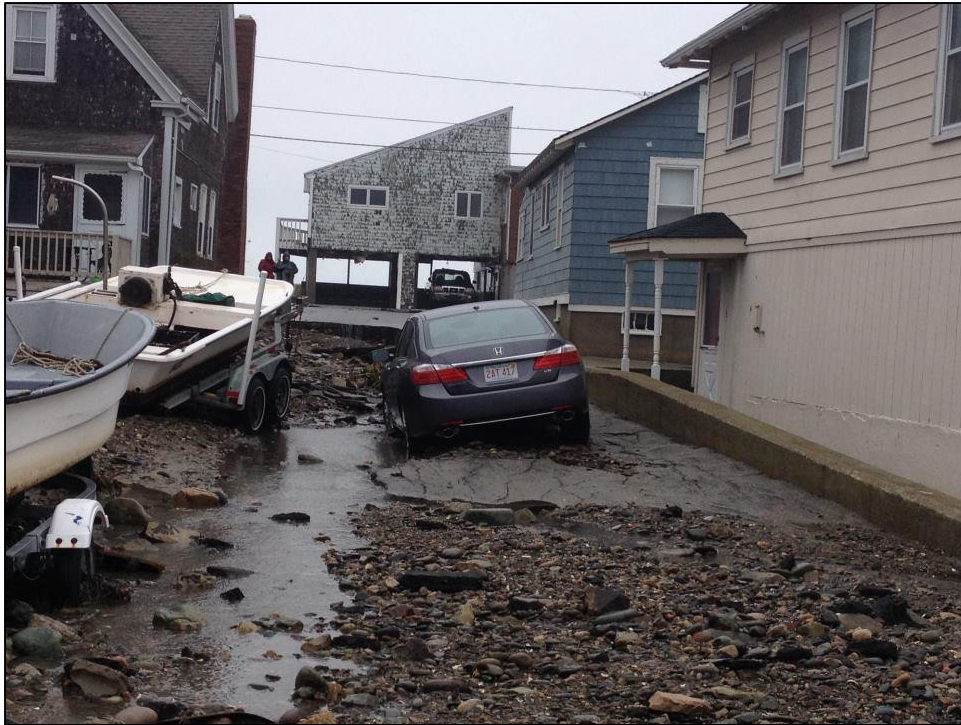
Figure 1.4. Damaged asphalt and overwashed sediment and debris after a minor storm on October 23, 2014 (photo from the Town of Hull).
