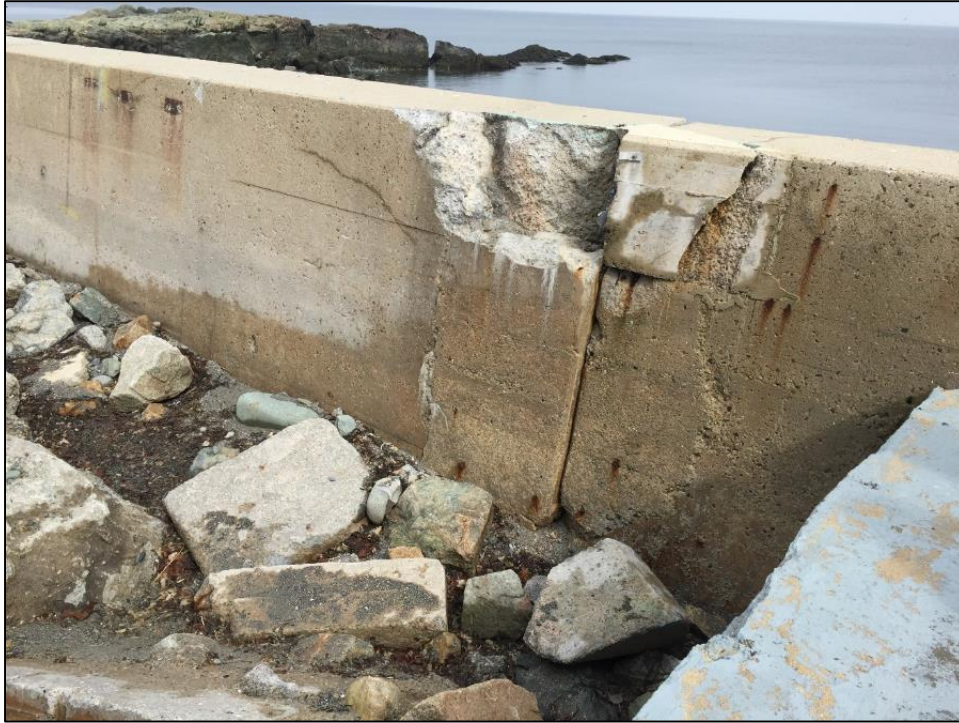
Figure 2.2. Spalling, cracking and breakage of the existing seawall (photo by Applied Coastal – March 26, 2015).
