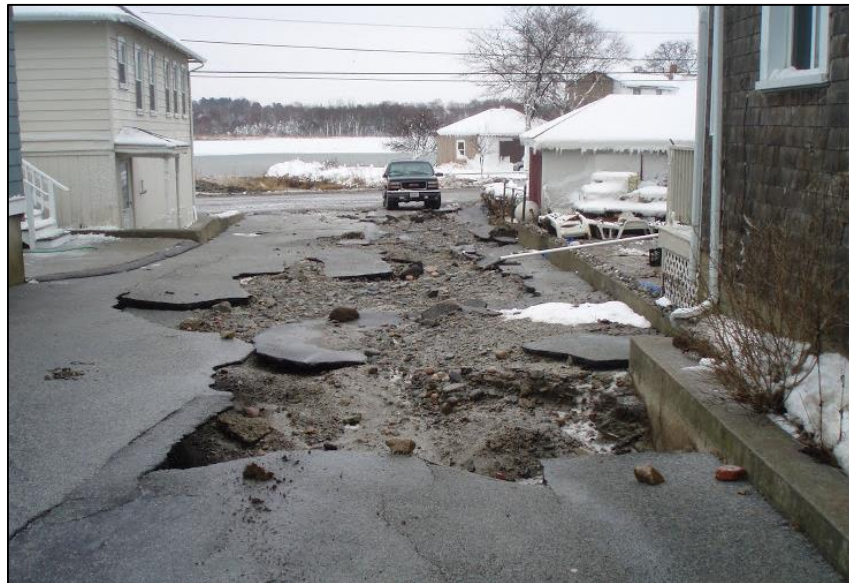
Figure 3.2. Damage to asphalt caused by wave overtopping and overwash (photo from the Town of Hull).
