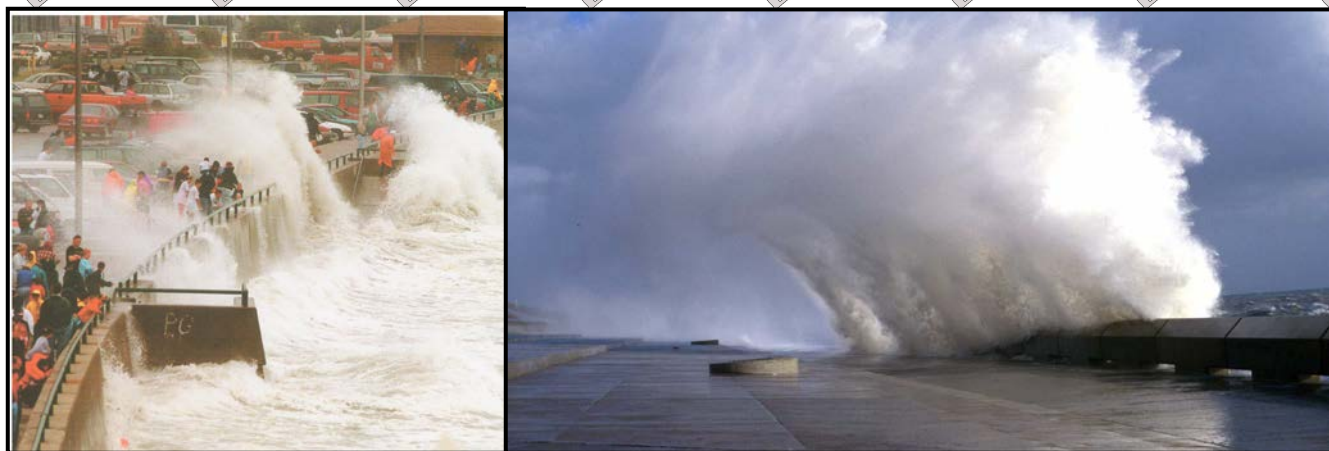
Figure 7-4. Examples of wave overtopping at seawall structures.
