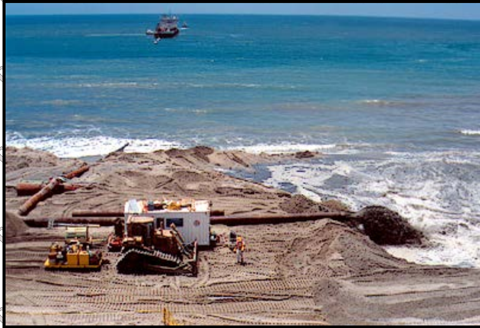
Figure 6-1. Beach nourishment project under construction.
