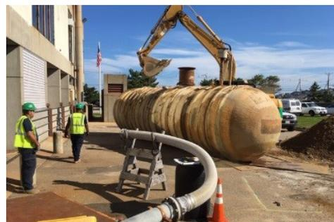
**Fuel storage tank after it was removed from the ground—no soil or groundwater contamination was found.**
