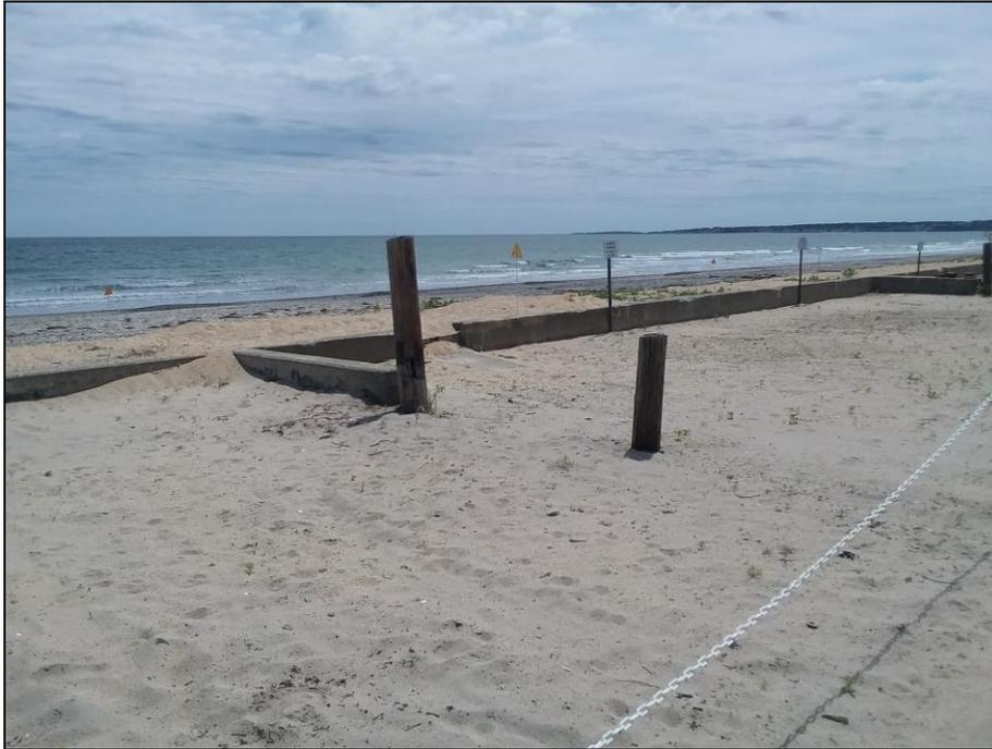
Figure 12. View of low-lying concrete wall, concrete separator walls, and wooden posts.
