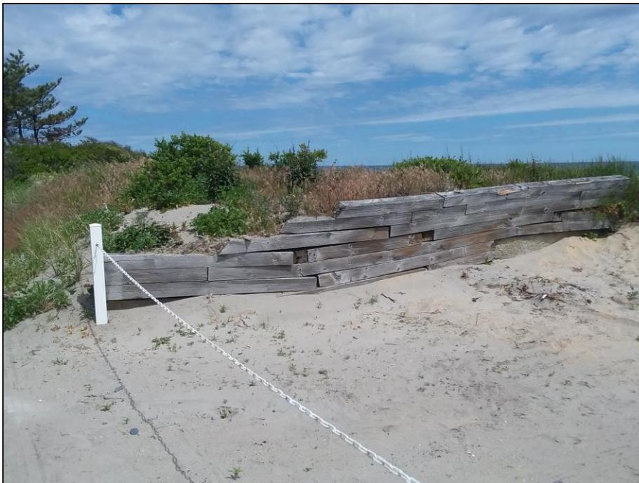
Figure 13. Photo of dilapidated timber retaining wall along the northern boundary of the project site.
